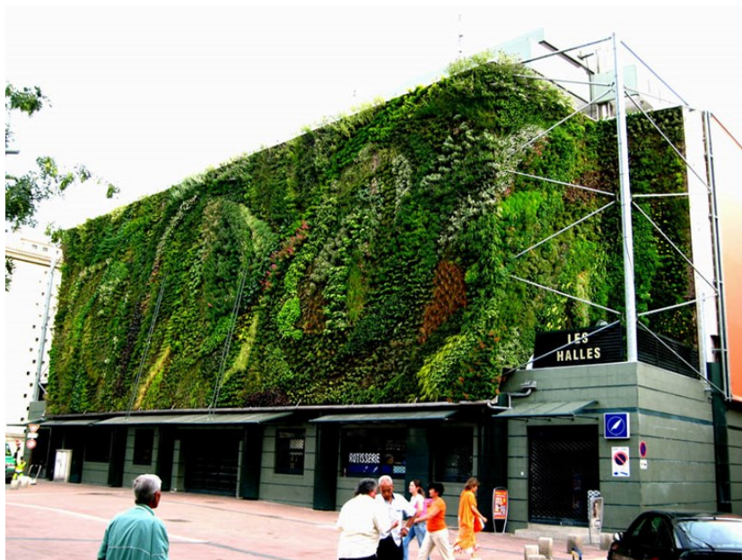
PHOTO 1. THE HALLES D'AVIGNON SHOPPING ARCADE IN AVIGNON, DESIGNED BY PATRICK BLANC
